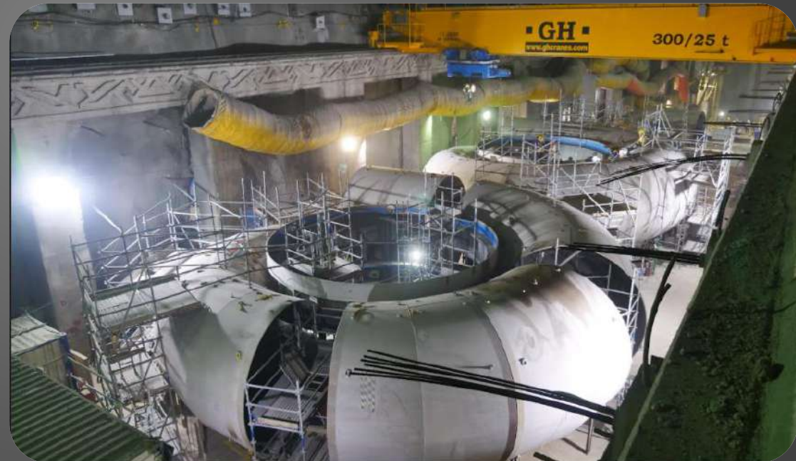
Powerhouse: Assembly of the first two turbines
