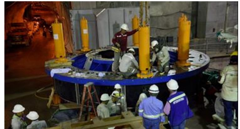
Civil Works at the Powerhouse: equipment's assembly (turbines and generators)
