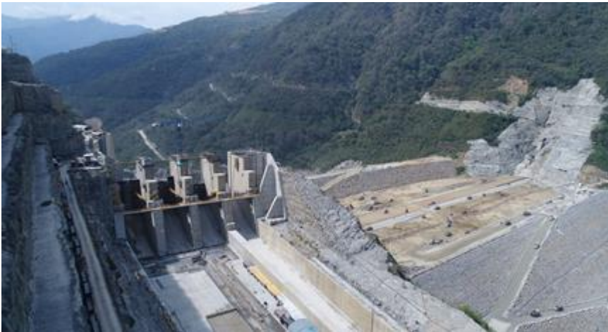
External civil Works: Spillway and dam
