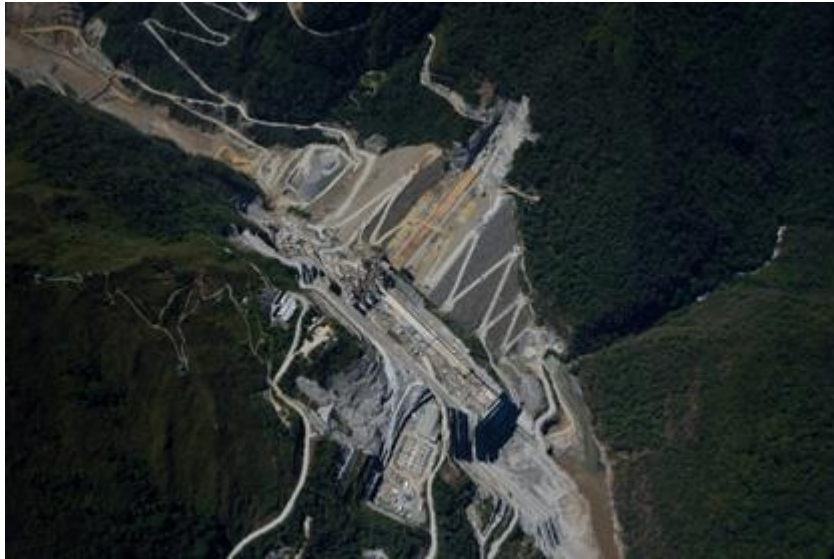
External civil works
