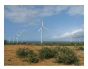
Implementing two wind farms with 200MW and 400MW generation capacity at La Guajira, integrated to the National Interconnected System I – SIN.
