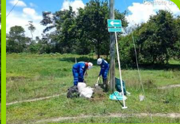
Installation of evacuation route signs.
