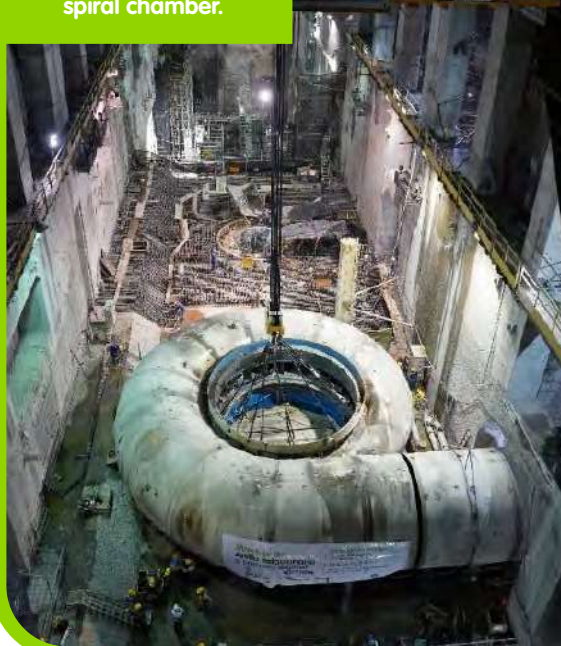
Stationary ring and spiral chamber.
