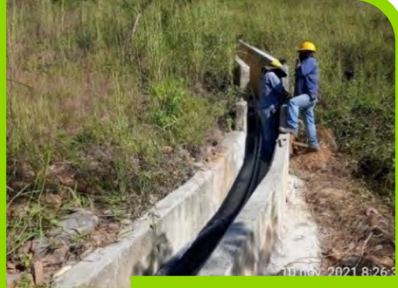
Repair of drainage works in revegetation areas.
