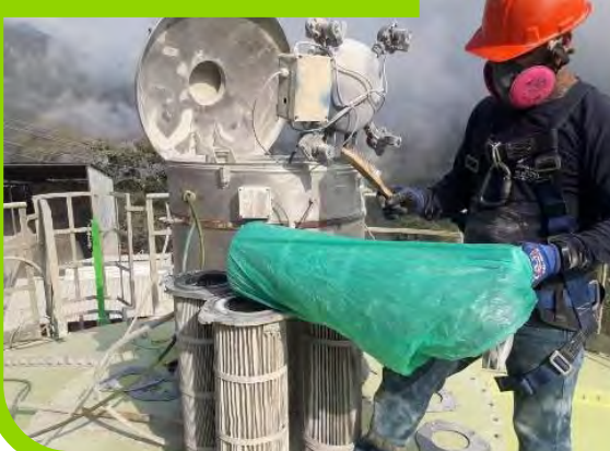
Cleaning of filters in cement storage silos.
