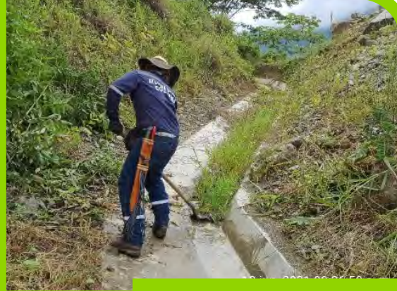
Cleaning of hydraulic works for the drainage of rainwater and runoff.
