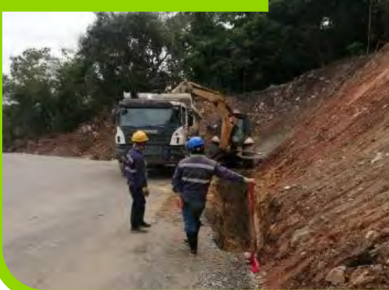
Construction of ditches for surface water treatment.
