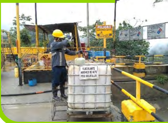
Preparation of anionic flocculant for the treatment of non-domestic wastewater.
