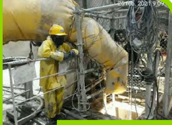
Implementation of ventilation system for confined spaces.
