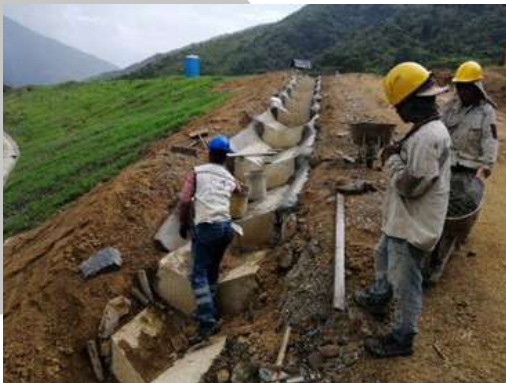
Formation of ditches for surface water treatment
