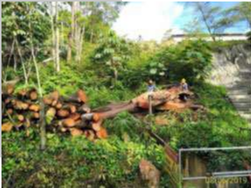
Chopping and temporary storing of trees close to felling sites
