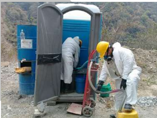
Cleaning of portable sanitary units' km 19 + 990
