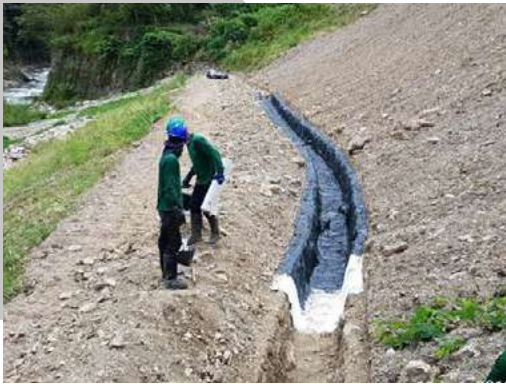
Drainage works in polymeiz material
