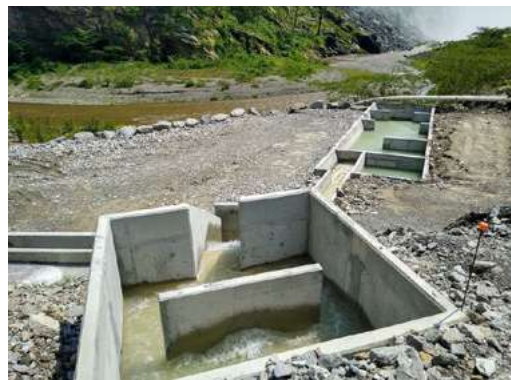
Sedimentation system for non-domestic wastewater treatment
