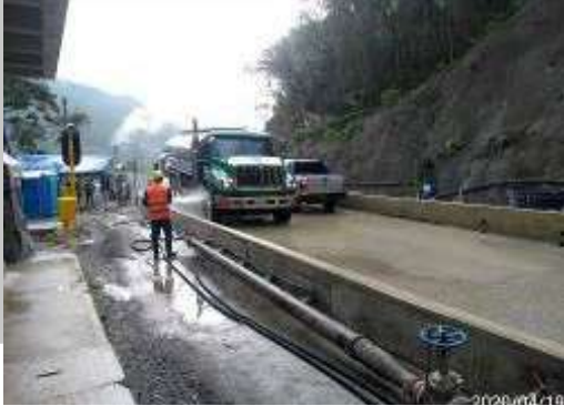
Washing vehicle tires entering paved roads
