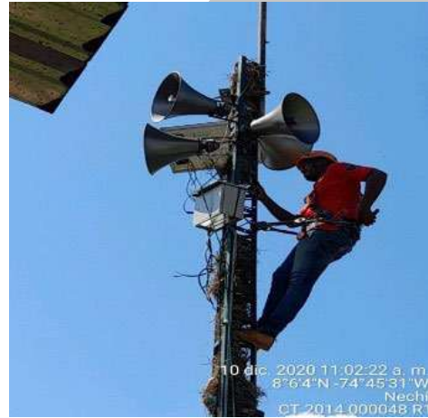
Alarm system maintenance work - Nechi
