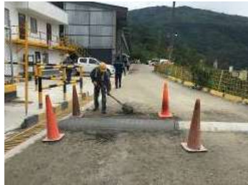
Construction of a speed bump to reduce vehicle speed
