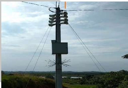
SAT Maintenance - Caucasia
