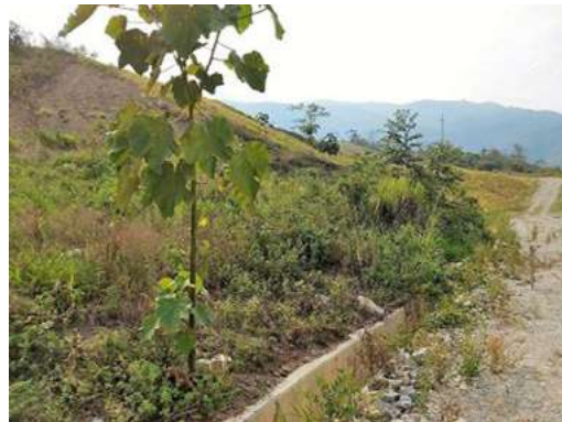
Concrete drainage and revegetation
