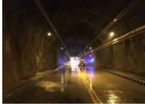
Tunnel track washing
