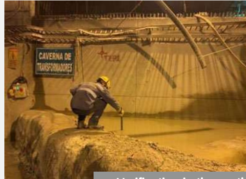
Verification in the north upper construction gallery
