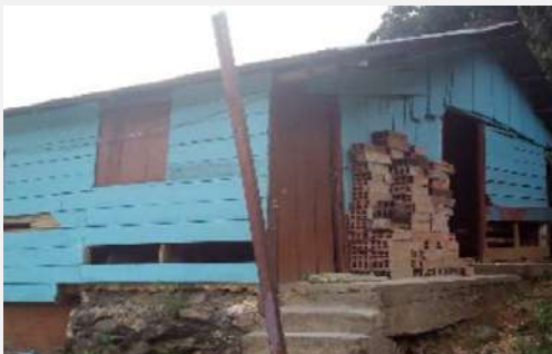
House in the Remolinos sector, built with unconventional materials (wood board walls, cement floor, zinc roof, bathroom with latrine, kitchen, and bedroom), with promissory purchase document, and located on a risky area.
