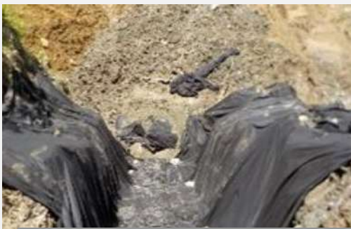
Construction of underground drainage filters for disposal areas
