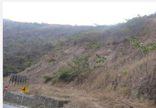
Gabions to control unstable site
