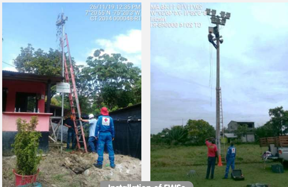
Installation of EWSs
