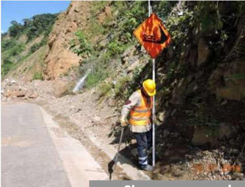
Signage on roads
