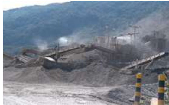
Particulate matter handling in the crusher
