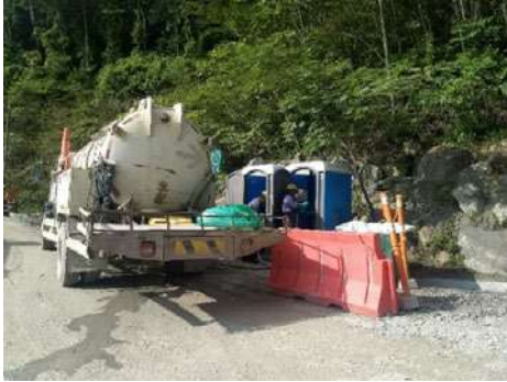
Cleaning of portable toilets with a Vactor truck
