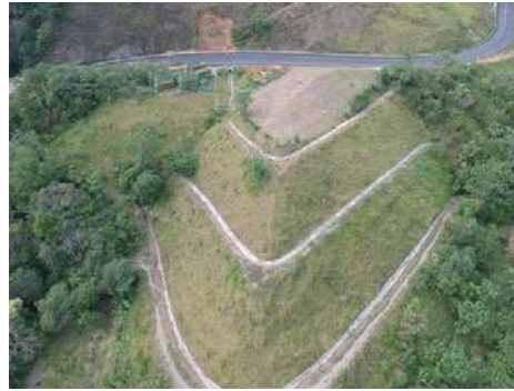
Disposal area with berms, ditches, and revegetation
