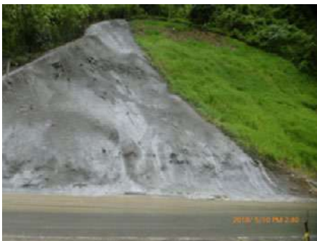
Shotcrete and revegetation combination for slope stabilization
