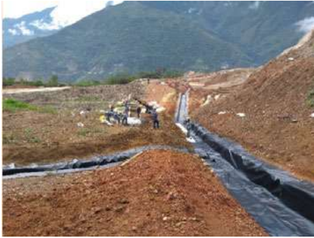
Construction of canals at the El Palmar materials source
