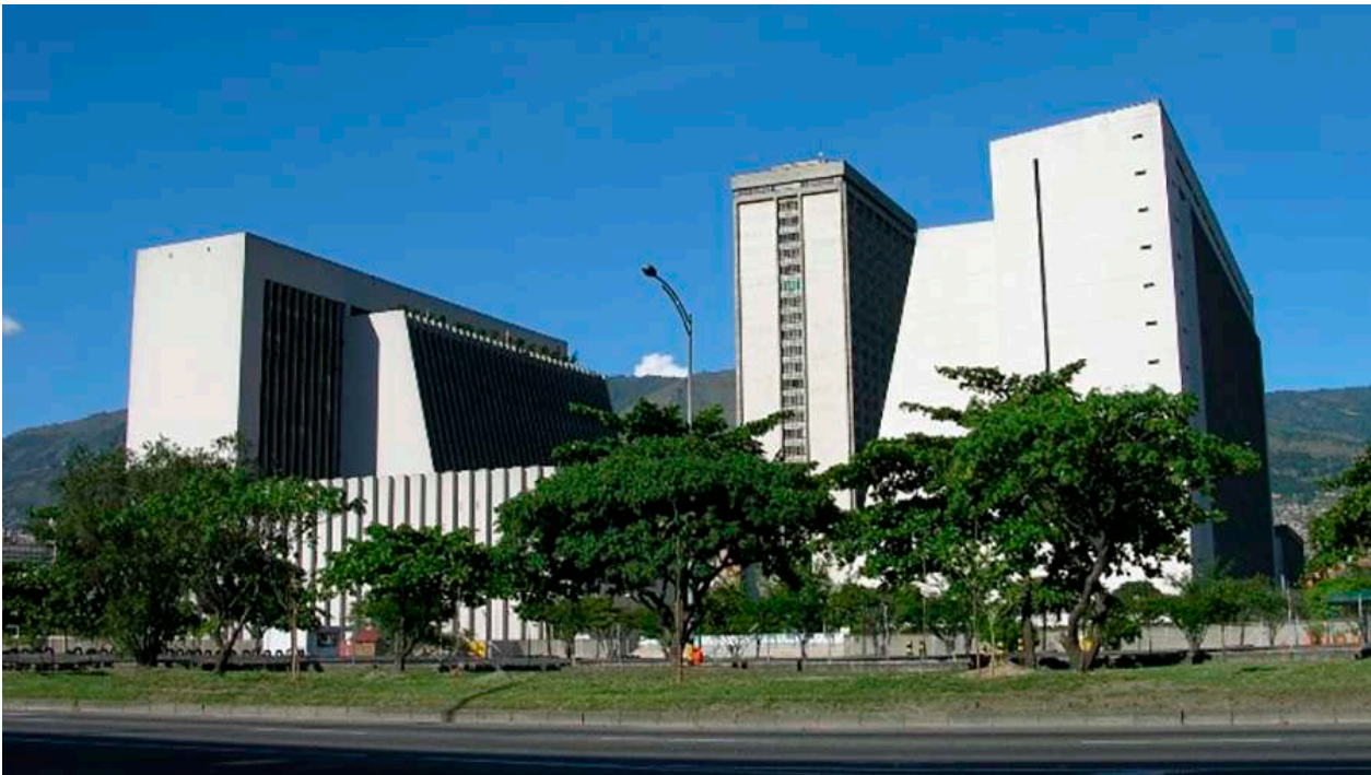
La Alpujarra Administrative Center. Urban building complex where the official headquarters of the Medellín Mayor's Office, the Medellín Council and the Antioquia Governor's Office are located.
