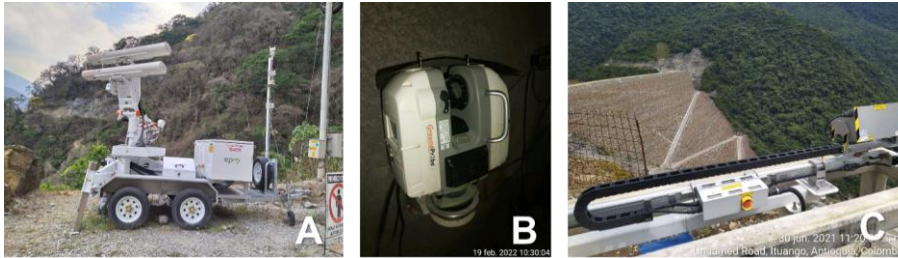
Figura 2-51. (A) Radar SSR528-FX, (B) GML, (C) Radar SSR410-SARX.
